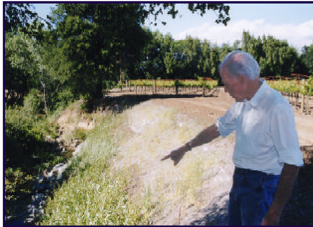
Quivira's Henry Wendt explains how they regraded stream banks to help restore Wine Creek as a spawning destination for returning salmon.
